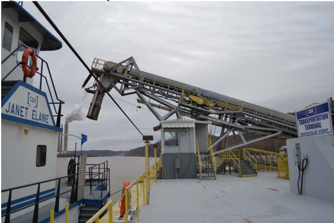
Figure 4: Coal Dock Facility
