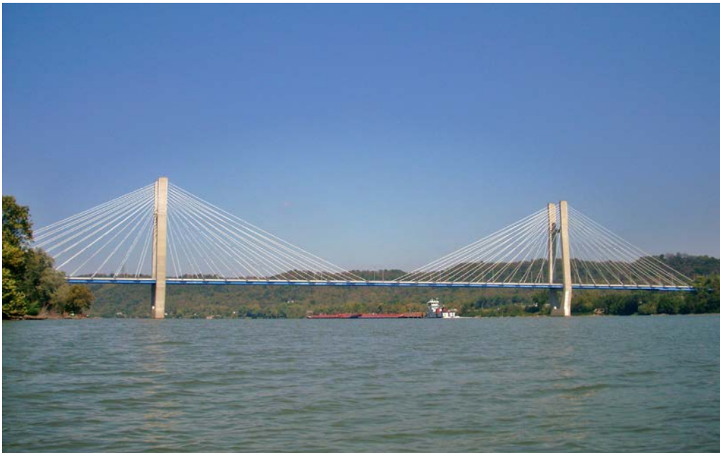
Image: William H. Harsha Bridge Maysville, Kentucky
